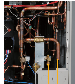
Liquid pipe Gas pipe
