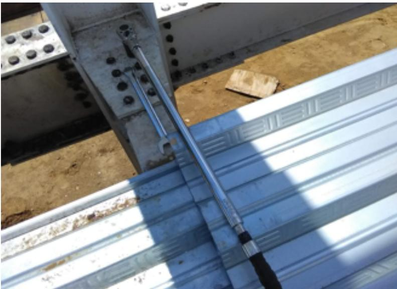
TORQUEO DE COLUMNAS Y TRABES METÁLICAS ENTRE EJES 1A -D, 2A- D, 3 A-D, 4 A-D Y 5 A-D.
