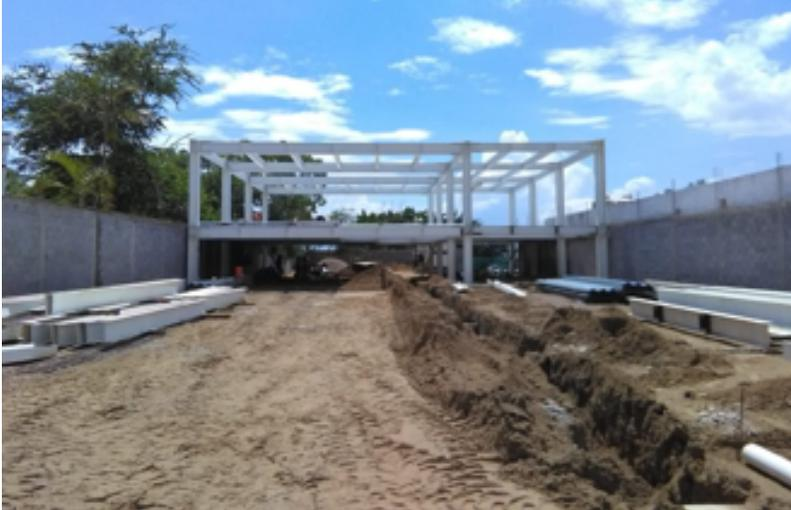
IZADO DE COLUMNAS Y TRABES METÁLICAS ENTRE EJES 1A -D, 2A-D, 3 A-D, 4 A-D Y 5 A-D; FALTANDO DEL EJE AL 9 TRAMO A-D.
